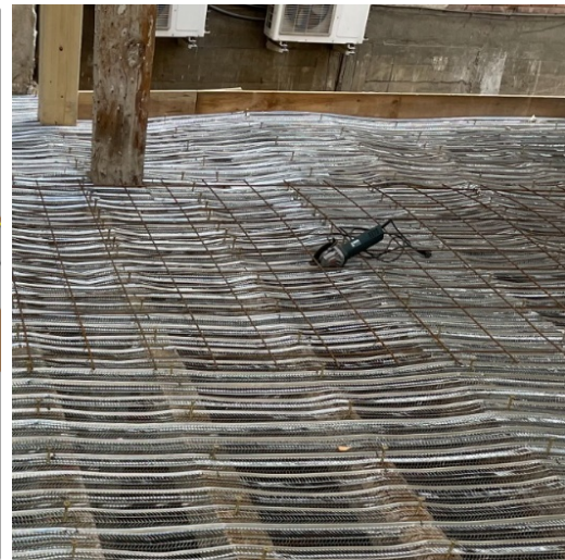
Figure 4: Laying of the mixed floor slab.
